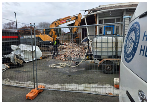
Demolition of old house behind Stanmore Rd Shop
